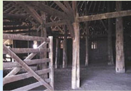
The Round Barn's interior structure.
