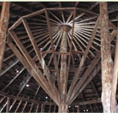
The barn's circular design is supported by a center truss-like structure.
